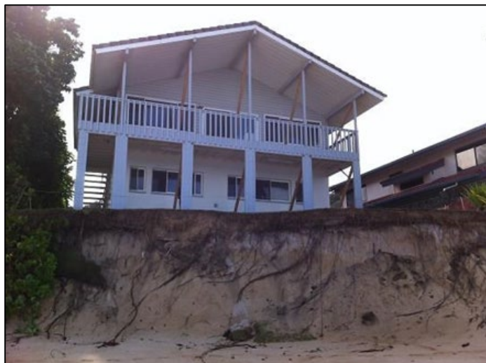
Figure 16. Beachfront home constructed on beach sand and threatened by severe coastal erosion at Sunset Beach, O‘ahu.
