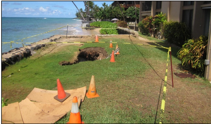
Figure 14. Example of a failing seawall and sinkhole caused by undermining from wave action and beach loss in West Maui (Tara Owens, Hawai'i Sea Grant).
