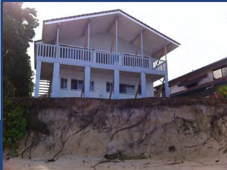
Figure 17. Beachfront home constructed on beach sand and threatened by severe coastal erosion at Sunset Beach, O’ahu.
