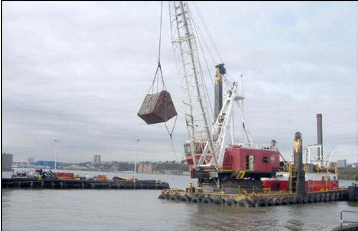
Figure 8-5. Clamshell dredge with environmental bucket
