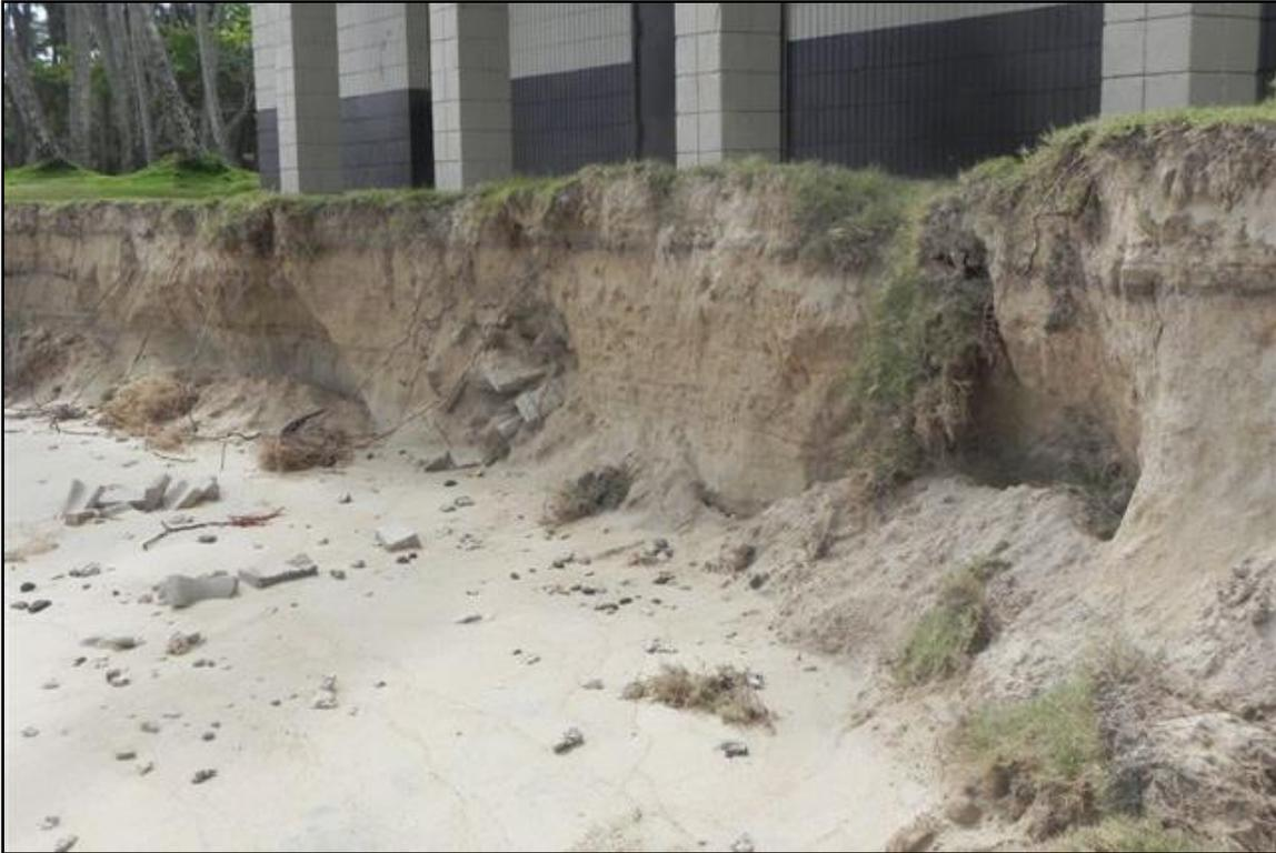
Figure 4-8. Erosion scarp at comfort station (winter 2015-2016)
