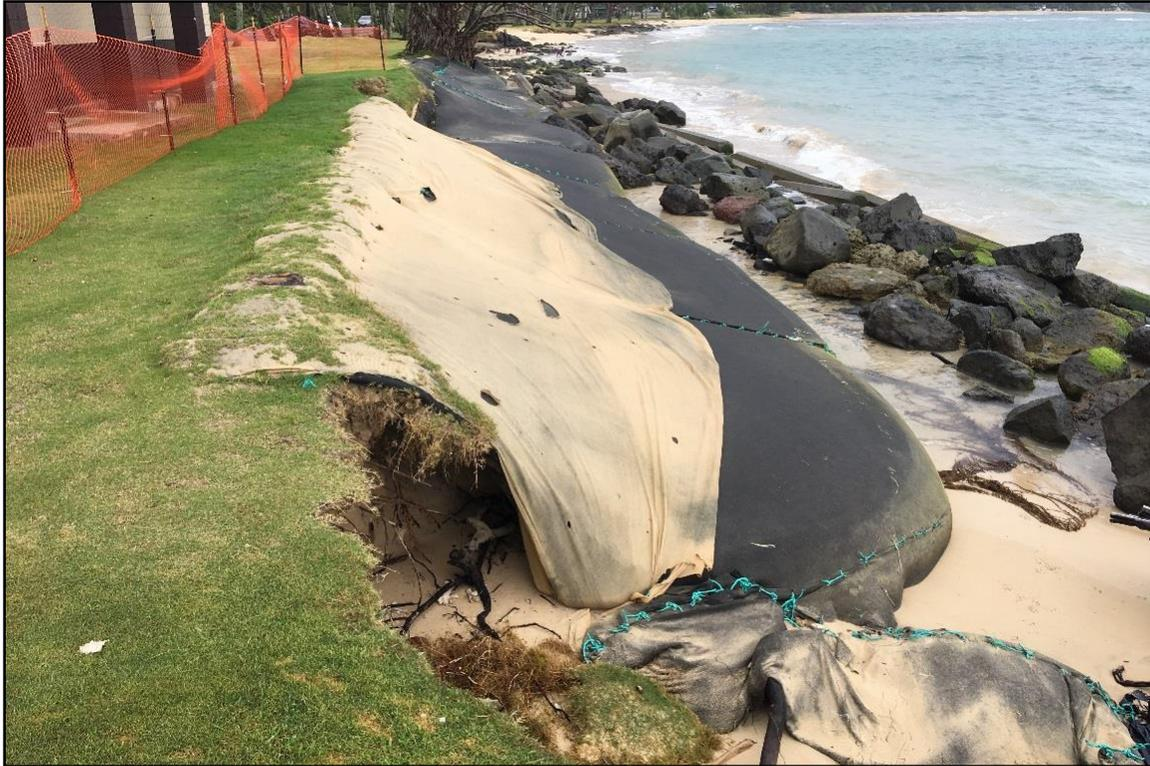
**Figure 4-10. Erosion protection fronting comfort station (January 2018)**
