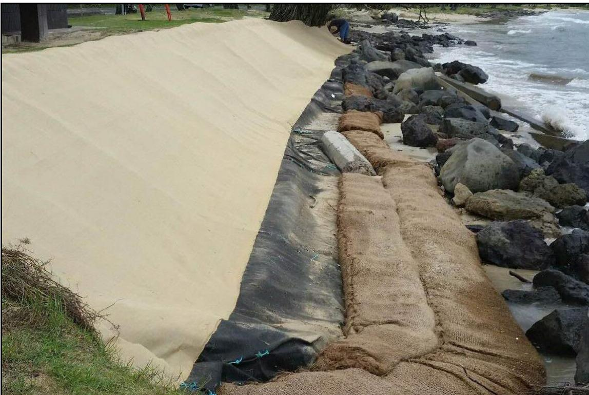
Figure 4-9. Erosion protection fronting comfort station (May 2016)
