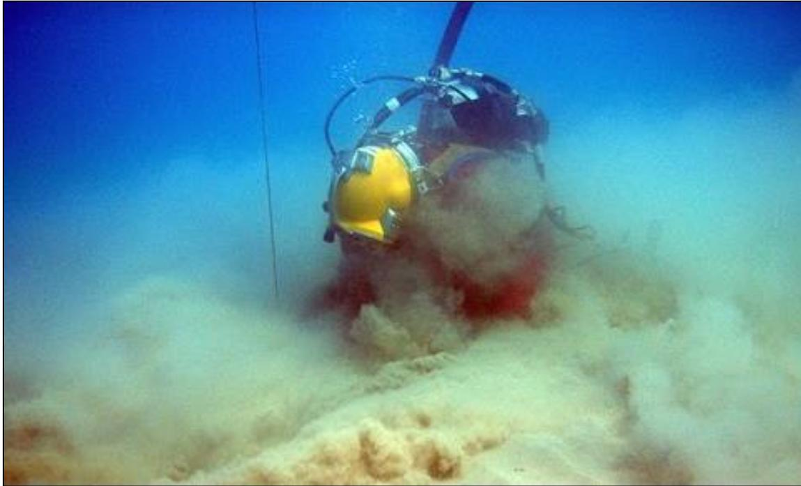
**Figure 8-2. Surface supplied air diver using a diver-operated dredge**
