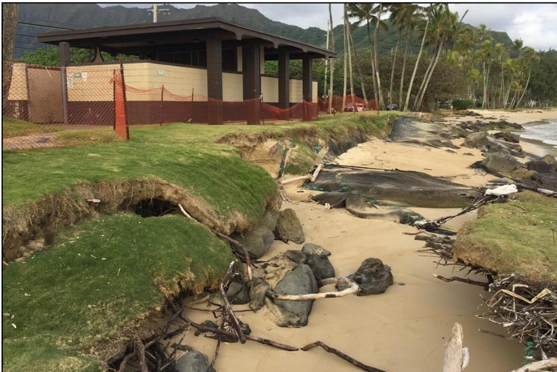
**Figure 4-11. Erosion protection fronting comfort station (March 2019)**
