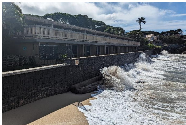
Kahana Sunset has experienced beach erosion that has rendered Building F uninhabitable, shown here in November 2023 (Photo credit L-R: EagleView CONNECTExplorer; SSFM)
