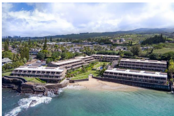
A historic photo compared with a recent photo shows the extent of beach erosion fronting the Kahana Sunset (Photo credit L-R: Kahana Sunset archives; Expedia).
